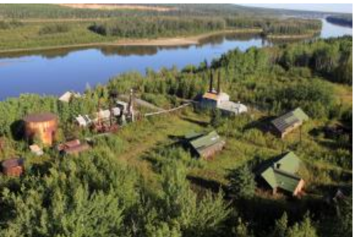
Facility operated from the '20s to '50s
